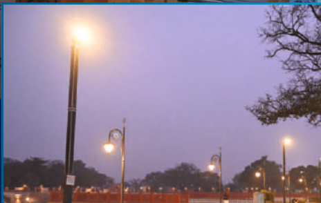
City lighting with Philips UrbanSpark, vertical solar panel integrated streetlight
