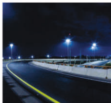
NHAI Street lighting
